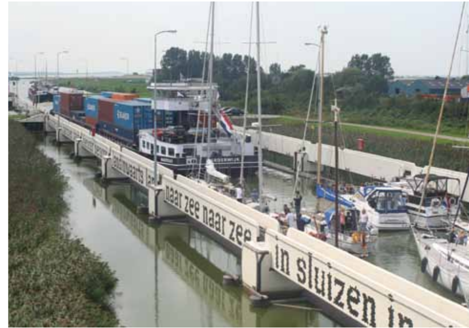
"Boaters can have problems in a lock when being flushed by a commercial vessel." Photo by Hylke Steensma
